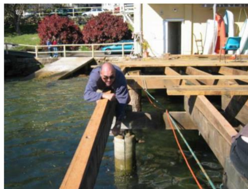
Current President Davis Lewis, tightening a few bolts on the wharf prior to the pontoon project
