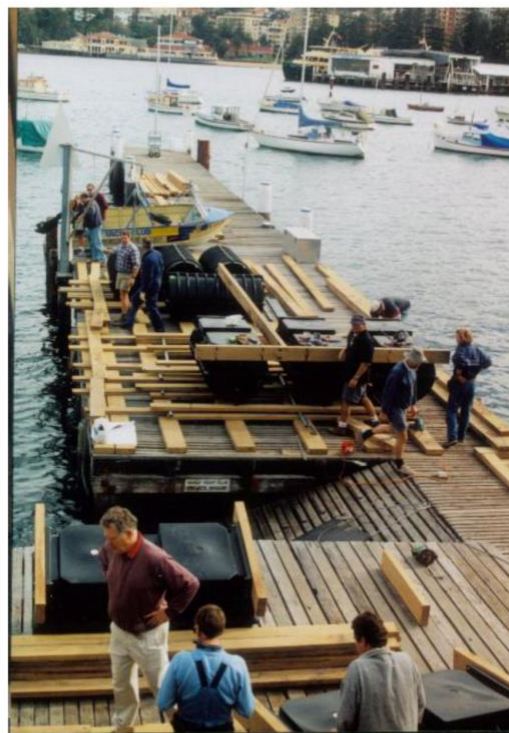
Assembly of the pontoon on the wharf
