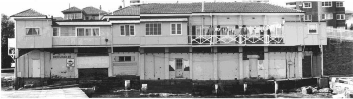
The old baths building being used as 2 flats just after the storm of 1974
